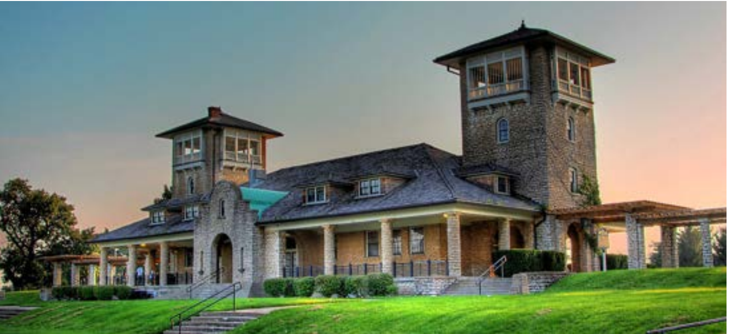
Figure 4.11: Former Swope Interpretive Center
